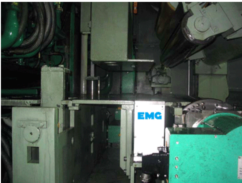
Fig. 5: Installed VKI sensors
